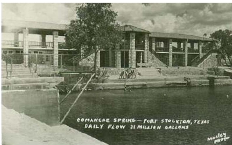
Figure 3. Photo of Comanche Spring pool before the spring ceased to flow. The estimated daily discharge was 21 Mgd.
